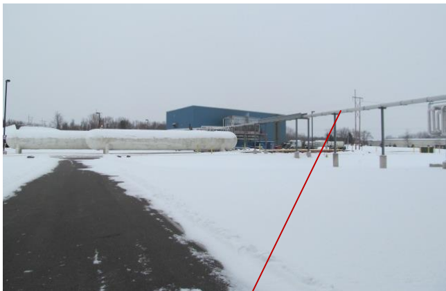
These pipes take carbon dioxide from the fermentation area to the building where it is bottled for use in soda pop.
